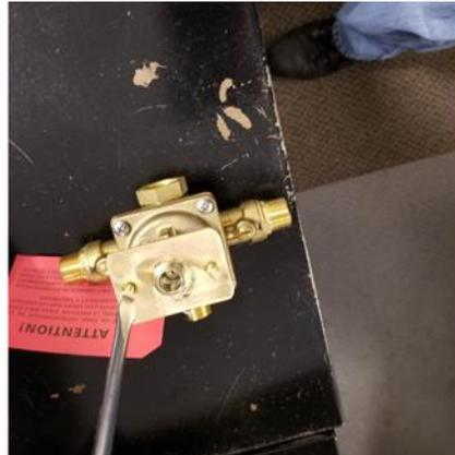
4. Take #4 bell and ensure #9 stem is inserted into the back of #4 bell as shown below left. Insert the assembly through the center of #1 mounting plate and fit it onto the rough nipple. Now finish screwing #2 slotted screws down tight to secure mounting plate to rough. (This aligns bell & stem.) Remove #4 bell & #9 stem and set aside for next step:
