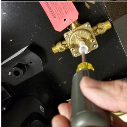
3. Take #1 mounting plate and place over center of rough with counter-sink holes facing up. Thread two #2 slotted screws into plate and leave them slightly loose:
